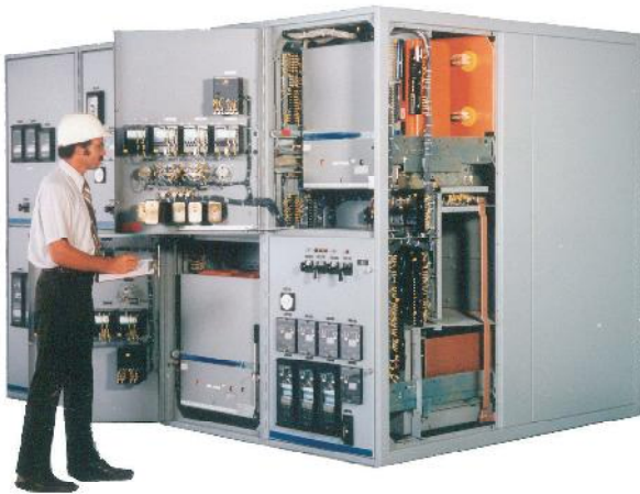
PACS engineers customize Metalclad Switchgear with a focus on safety and ease of access for maintenance.
